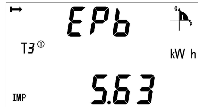
Current forward active energy on B phase
