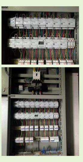
Project Overview: Client buy Acrel IoT EMS cloud system, hardware use ADF400L multi circuit energy meter, AWT100-CE ethernet gateway.
