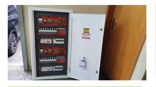
Project Overview: Isolation Power Supply System, hardware use AIM-M10, AIM-M100, AIM-M150, AIL150-8,AID150,AID200,AIM-R100,AKH-0.66P26 Project Amount: About \$720000
